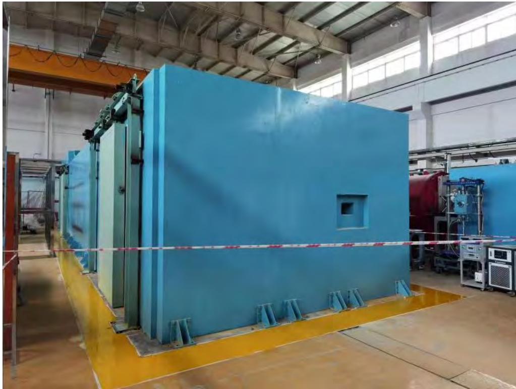
Big Shielding House is ready.
