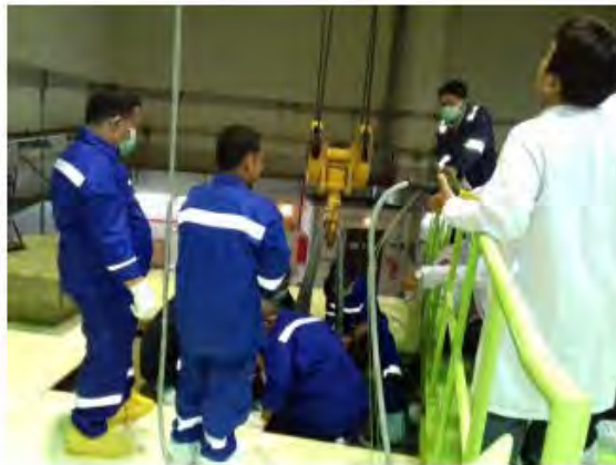
Beam tube: valve & shielding replacement
