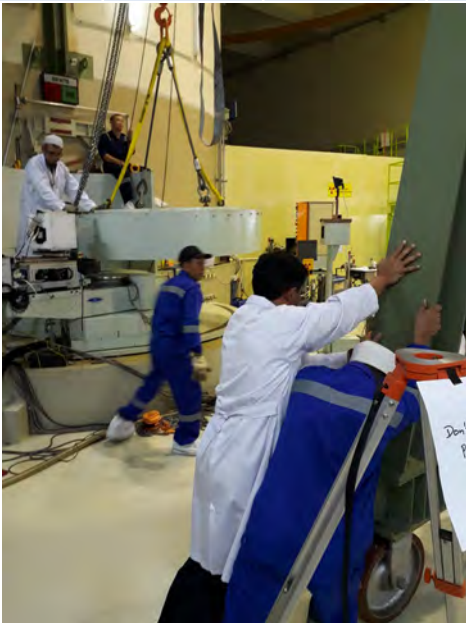
Repairment of shutter system of S6 beamtube
